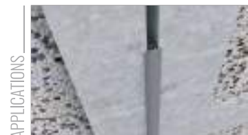
50 mm gap for stainless steel corner
